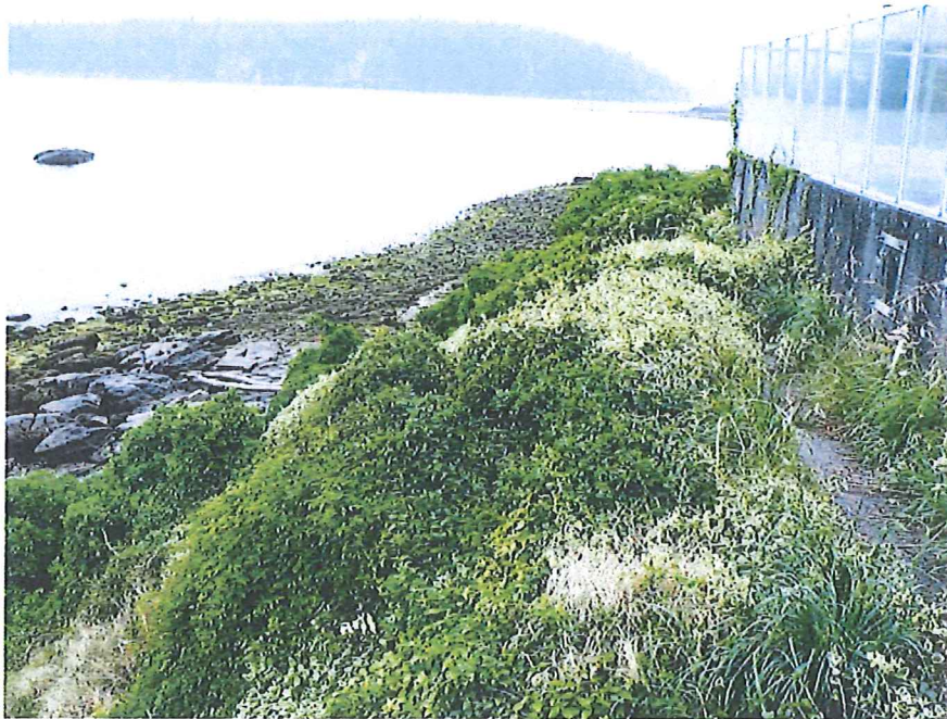
Photograph 4. View south to slope between natural boundary and pool wall.
